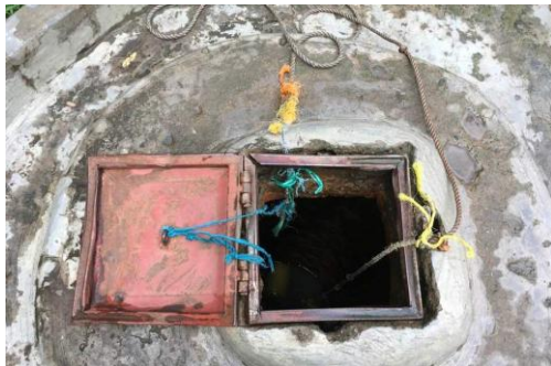
A water source in Kenya.
